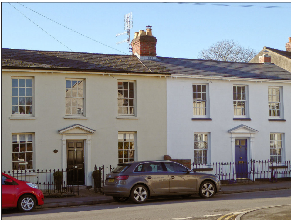
Figure 8: Early houses, Chapel Road
