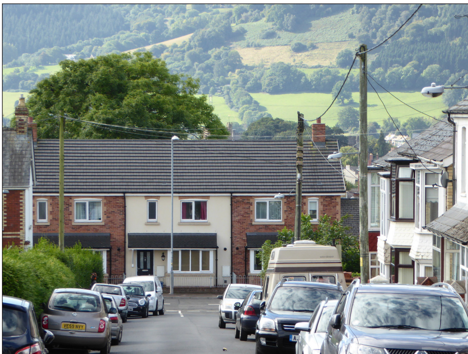
Figure 10: recent building, Grosvenor Road
